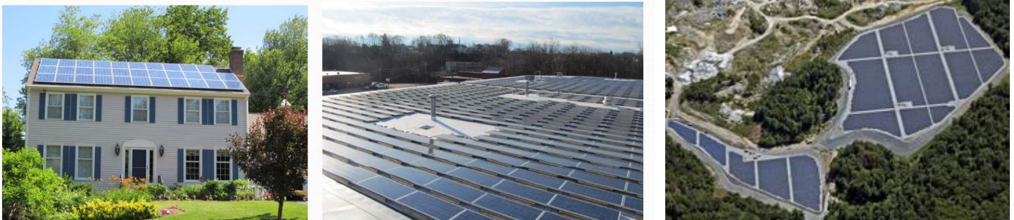
From left to right: Typical residential solar, small commercial and large commercial installation at Westford Solar Park. (Source: MassCEC and Cathartes Investments).
