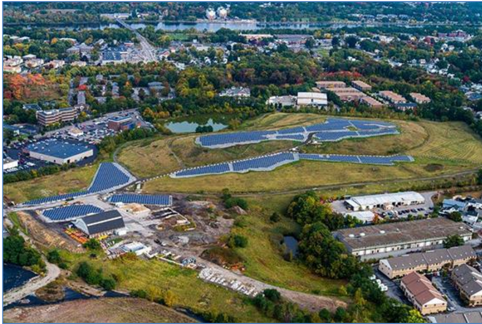
Exhibit 2: Lowell’s closed and capped landfill with solar array
